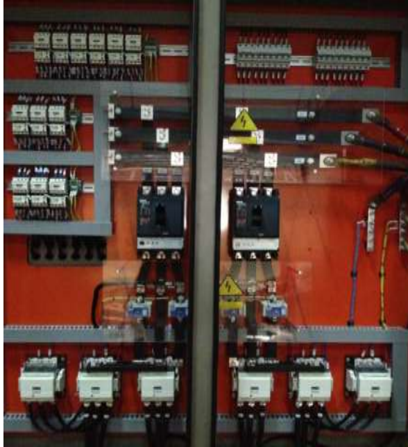
Starter high voltage side
