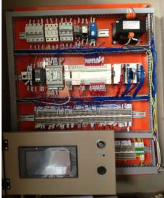
Control box low voltage side
