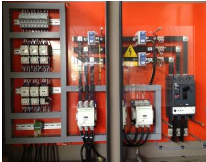
Starter high voltage side
