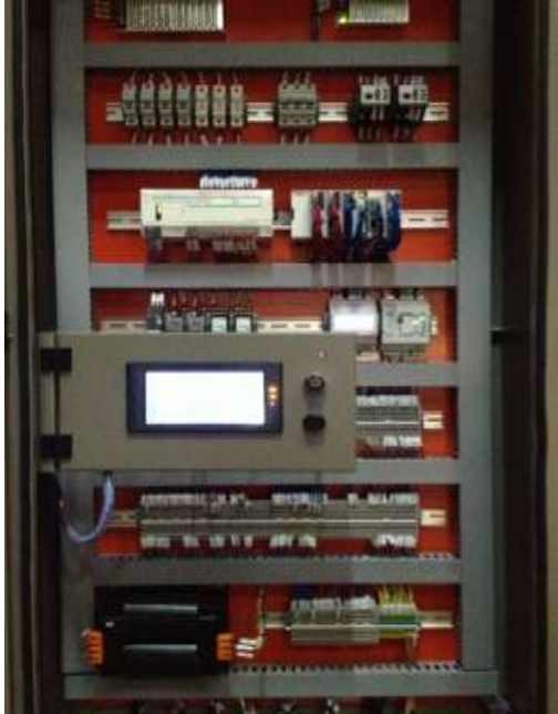
Control box low voltage side
