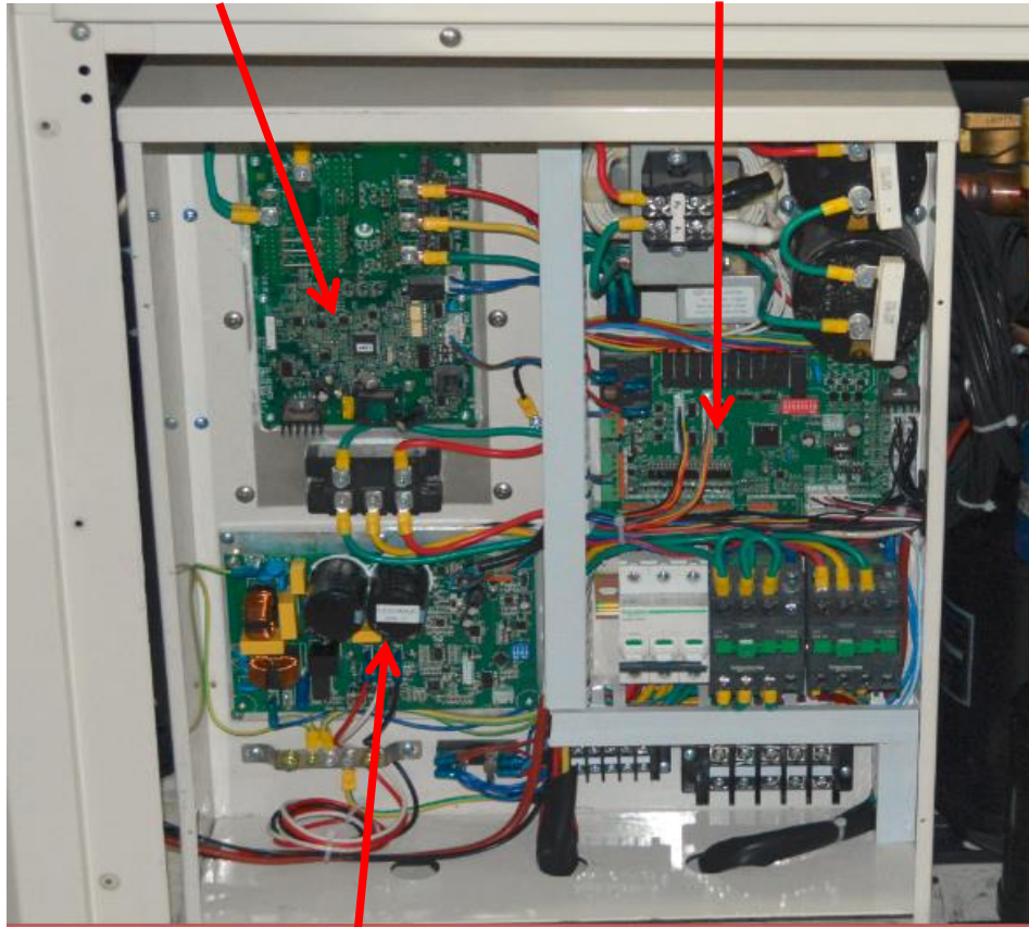
controller main PCB panel
